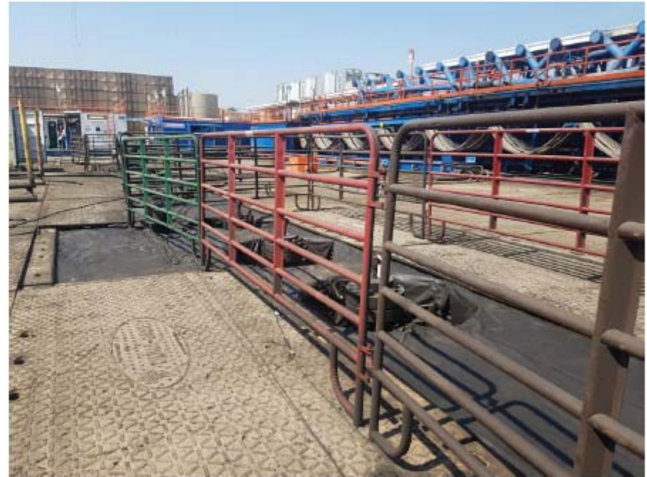
Extraction rig, September 2017
